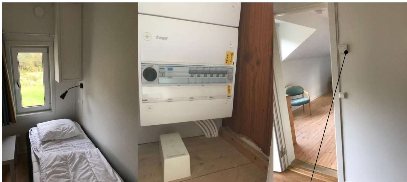
Central termostat 1 Tr
